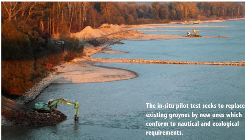
The in-situ pilot test seeks to replace existing groynes by new ones which conform to nautical and ecological requirements.
